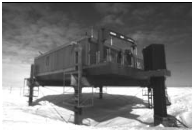
The Simpson building which houses the ozone laboratory at Halley Research Station. The people standing on the scaffolding are jacking the platform to stop it from being buried by drifting snow
