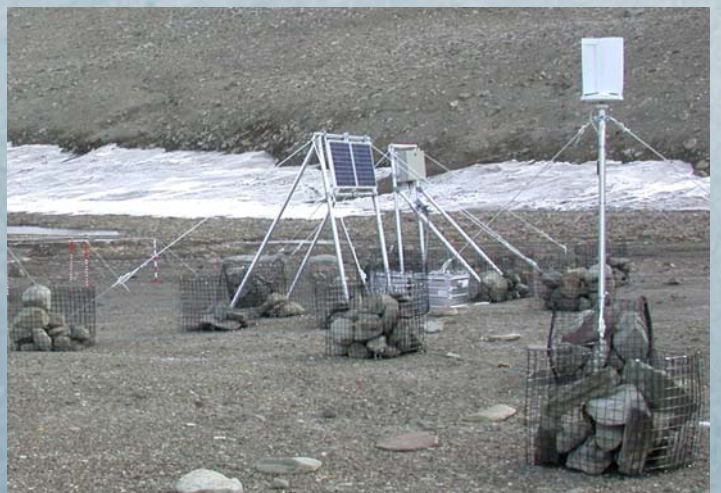
System at Mars Oasis. Wind generator, solar panels, camera and battery boxes can all be seen.
