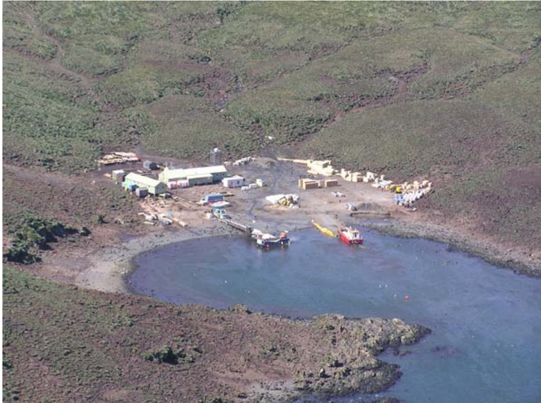
Transformation in progress, unloading the tender at the new aggregate jetty
